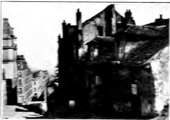
OLD BUILDINGS OF THIS SORT ARE BEING TAKEN DOWN TO BE REPLACED BY MODERN MUNICIPAL APARTMENTS
